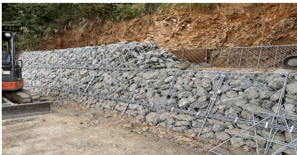
Figure 6.11 Gabion Check Dam
