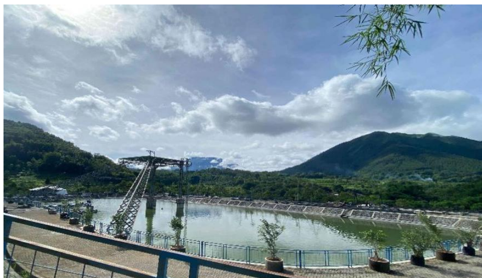
Figure 6.23 Application of Water Reservoir
