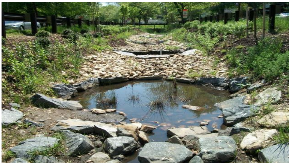
Figure 6.10 Loose stone Check Dam
