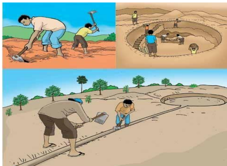
Figure 6.20 Construction of a Rainwater Reservoir (Source: Godinho et al. , 2023)
